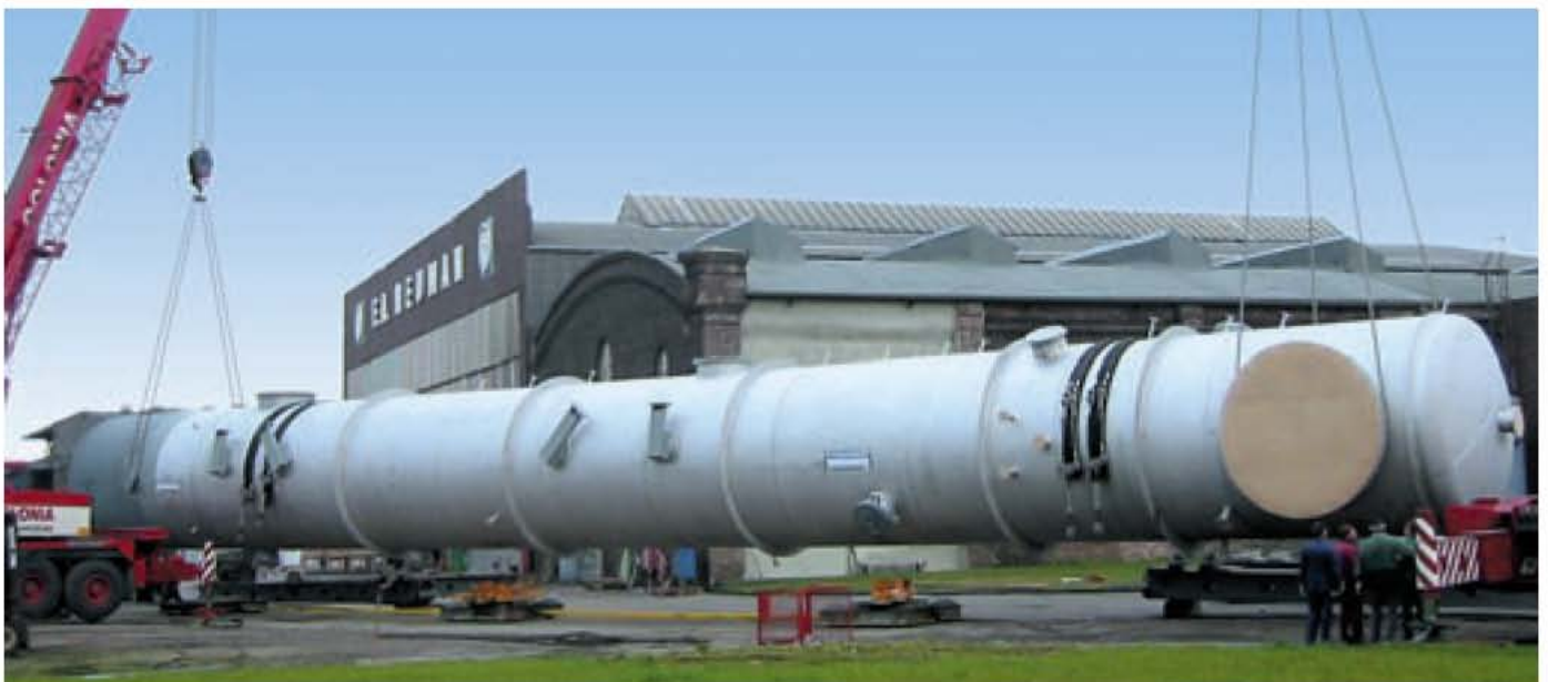
Dividing wall column DN 3600
